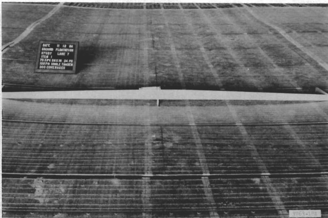
Fig 6. Lane 7, item 1. Transverse straightedge shows roughness at 300 coverages (failure)
