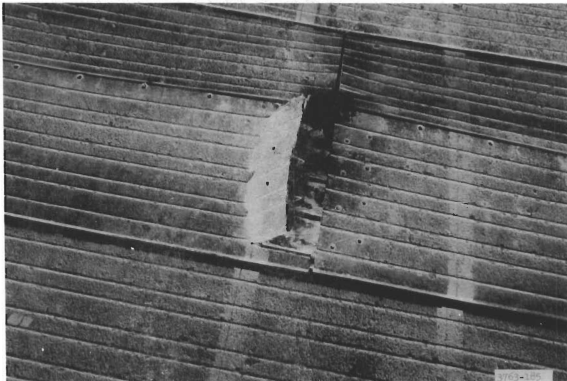
Fig 5. Lane 7, item 1; closeup view of severe mat break at 300 coverages (failure)
