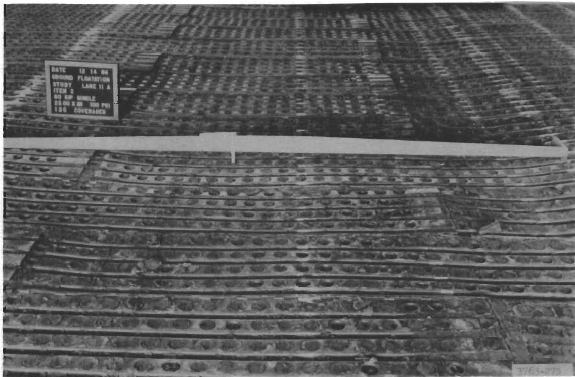
Figure 10. Lane 11A, item 2. Transverse straightedge shows deformations at 130 coverages (failure)
