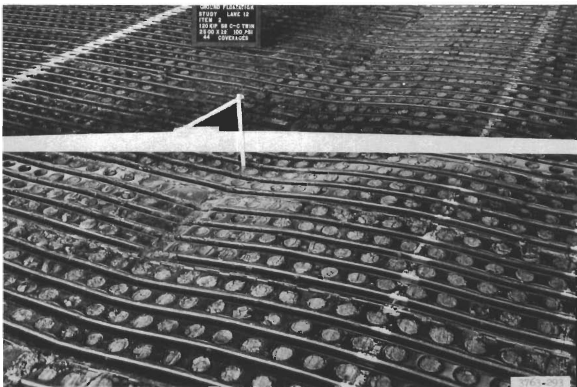
Figure 15. Lane 12, item 2. Transverse straightedge shows deformations at 44 coverages (failure)
