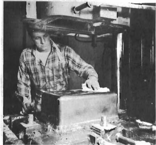
FIG. 20.041.1 POLISHING THE MALE HALF OF A MOLD PRIOR TO PLACING LAY-UP IN A PRESS MOLDING OPERATION (LUNN LAMINATES)
