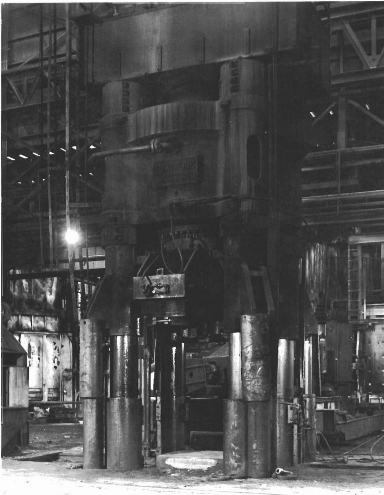
Figure 29. Hydraulic Forging Press Rated at 6000 Tons of Force and Employed by Cameron Iron Works, Inc., to Produce Fin Rib Forgings. Shown with Dies Removed. Note Gas-Fired Furnace Behind the Press at Right which was Used to Heat All Workpieces for Forging, and Large Manipulator on Rails Between Furnace and Press.
