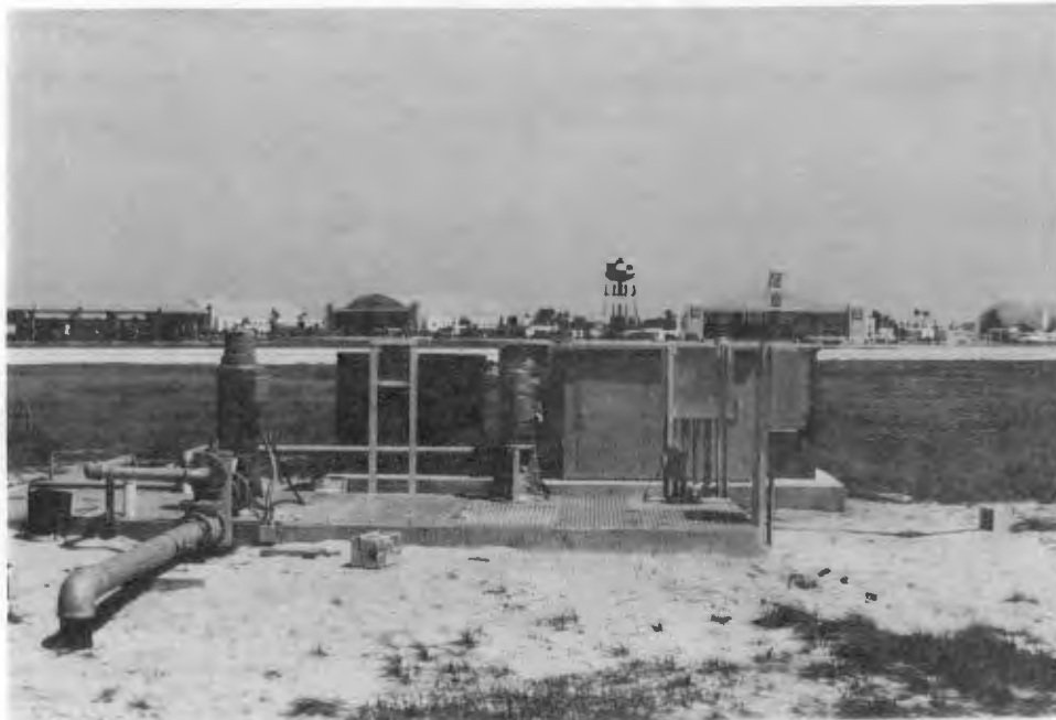
Figure 13. View of the USAF Automated Rinse Facility.
