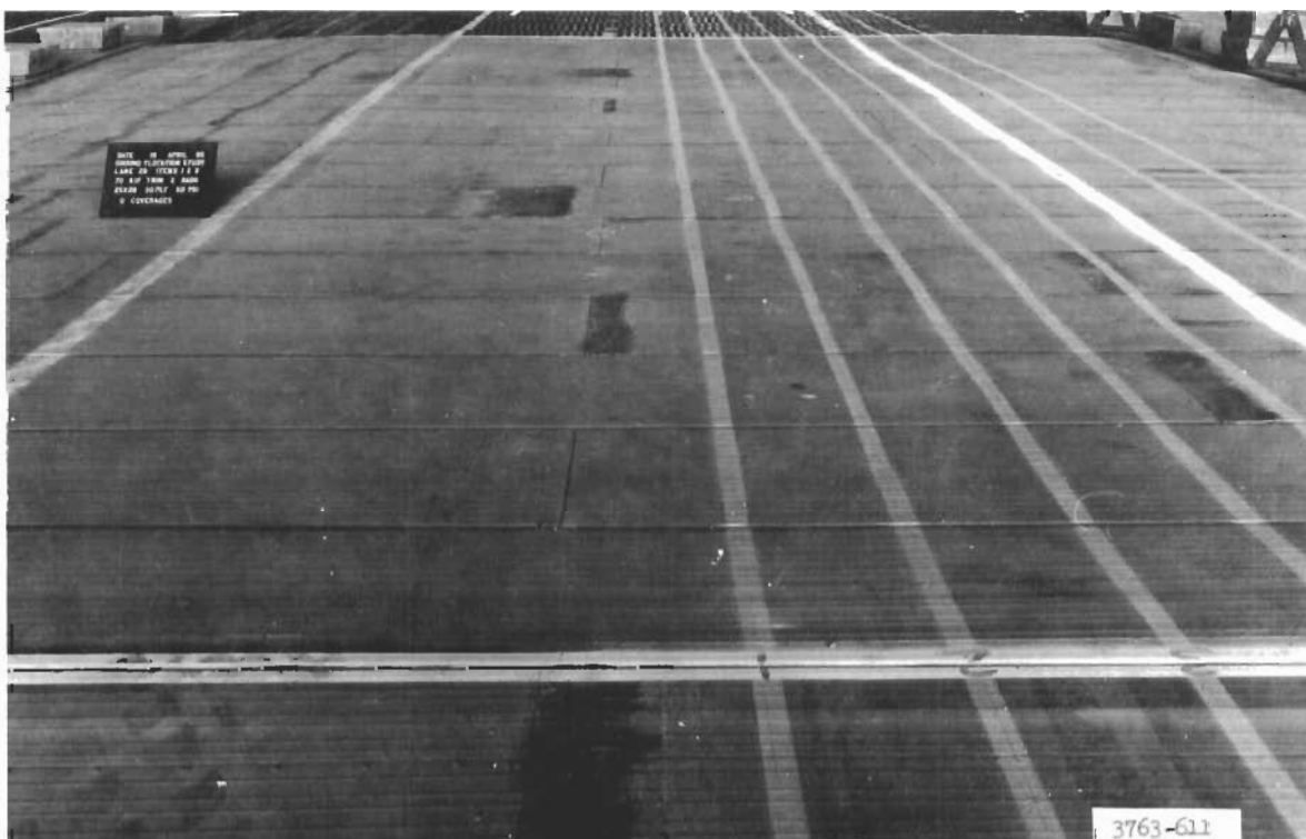
Figure 9. Lane 29, item 1, prior to traffic
