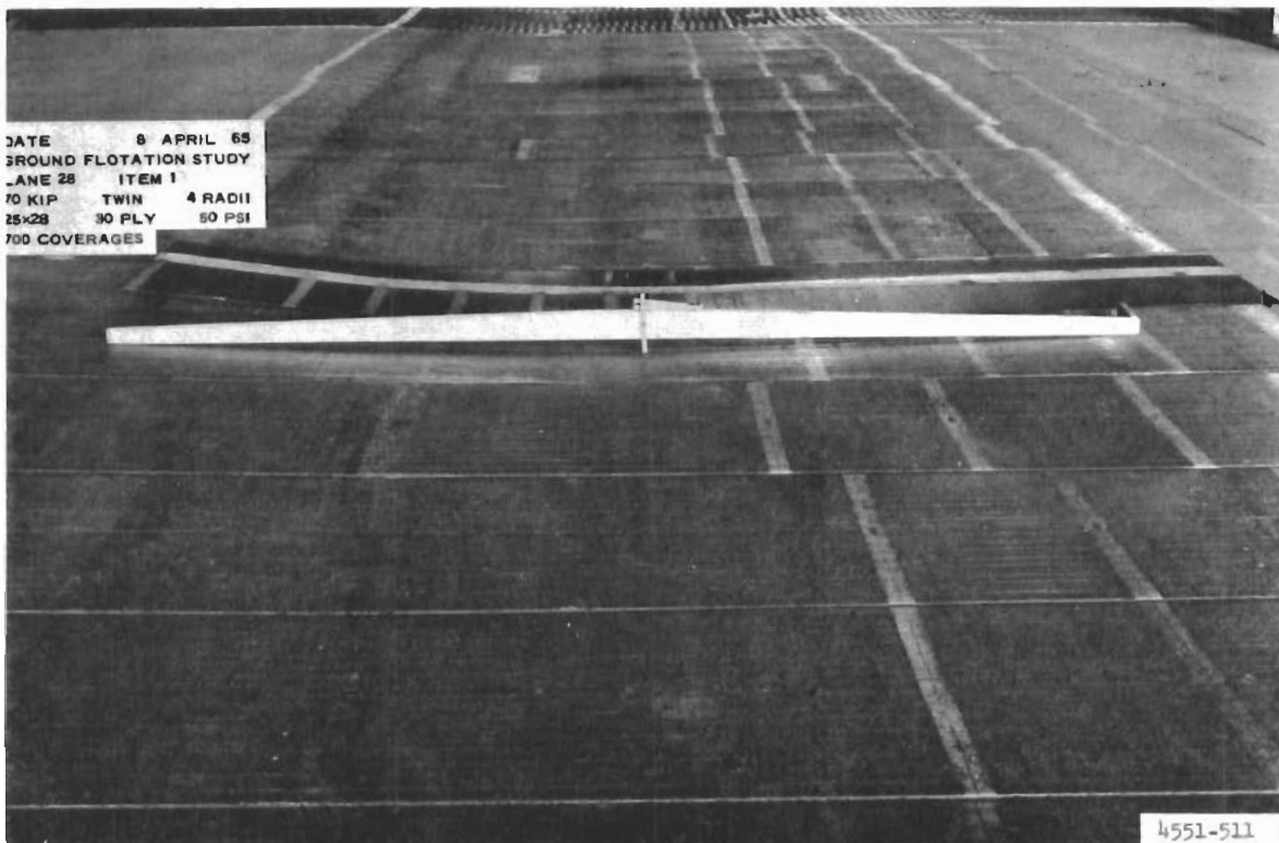
Figure 4. Lane 28, item 1, after 700 coverages of traffic (failure)
