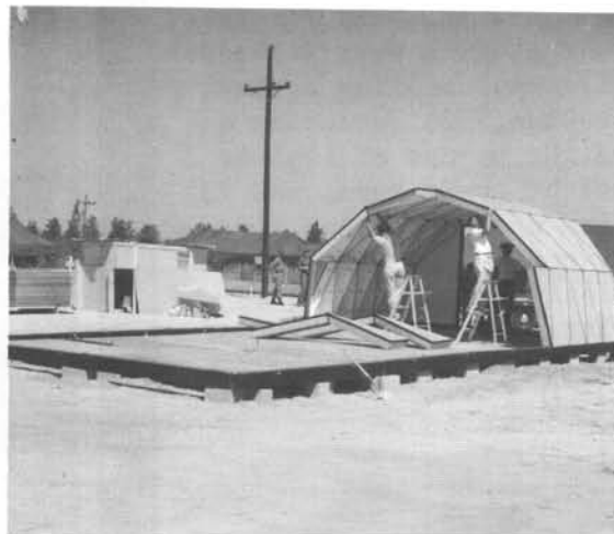
FIGURE 21. Shelter #1 - Erection at Eglin AF Base, Florida
