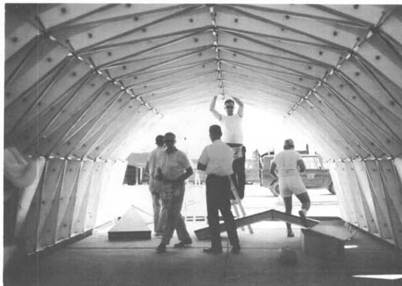
FIGURE 23. Shelter # 1 interior view during erection.
