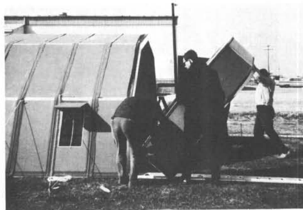
FIGURE 41. Shelter # 2. erection of "folded beam" arches, Langley AF Base, March 1965.
