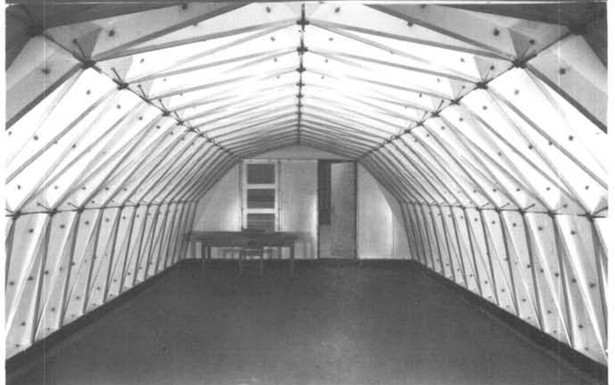
FIGURE 18. Shelter # 1 interior view.
