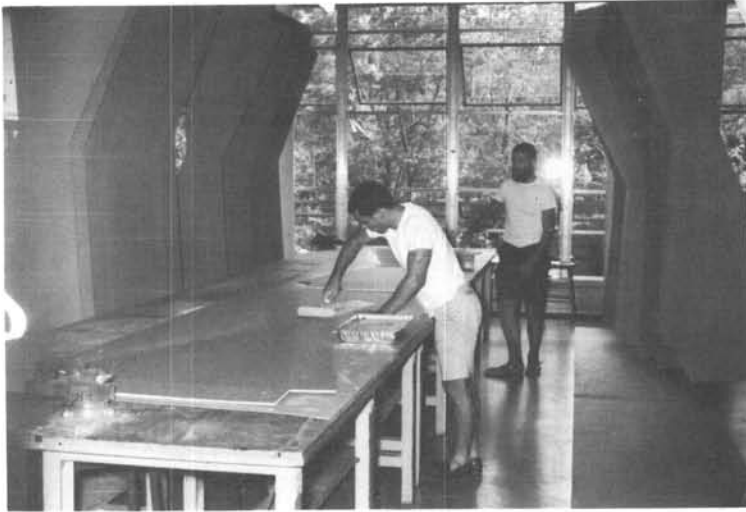
FIGURE 16. Production of Shelter #1. Application of epoxy-type coating.
