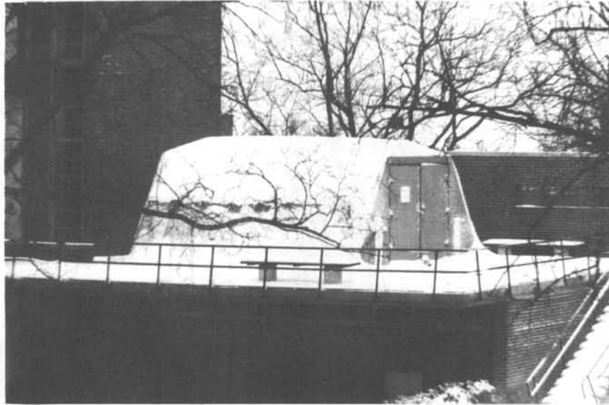
FIGURE 24. Shelter #1 Snow-load test at University of Cincinnati. February, 1965
