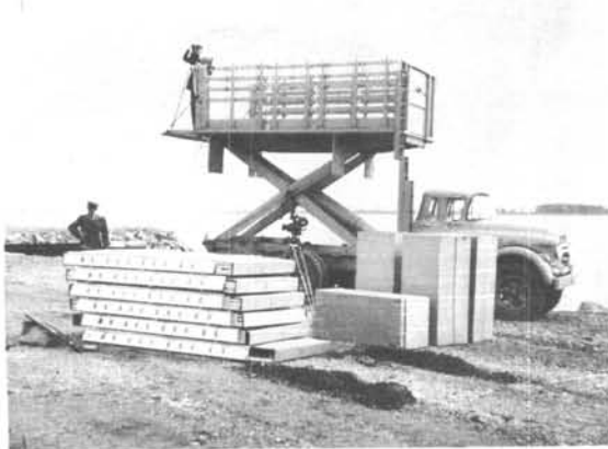
FIGURE 40. Shelter # 2. Langley AF Base, Va. Packaged Shelter left: basic shelter, right: insulation kit.
