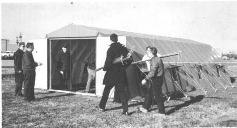
FIGURE 42. Shelter # 2 Erected shelter showing end with large doors.
