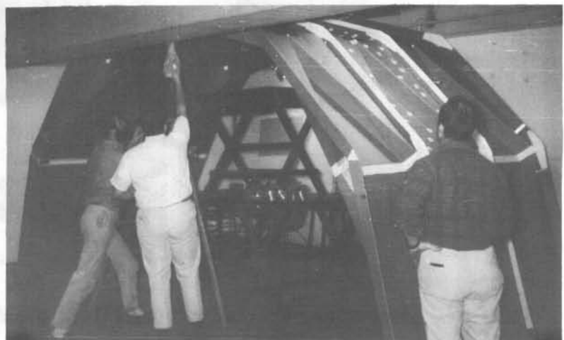
FIGURE 32. Test arch Fome-Cor "folded diamond" concept.
