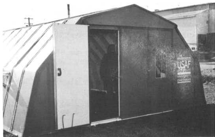
FIGURE 43. Shelter # 2 Erected shelter showing end with small door, filler panels.
