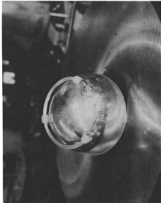
Figure 49. Vent Tubes, Upper Inner Shell
