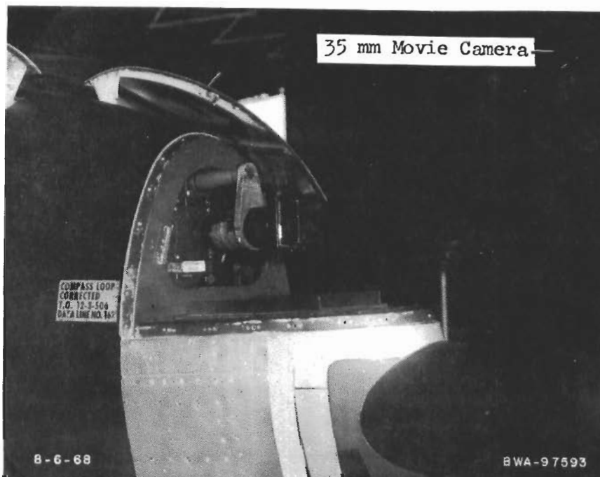
Figure II-1 Front View of Camera Installation
