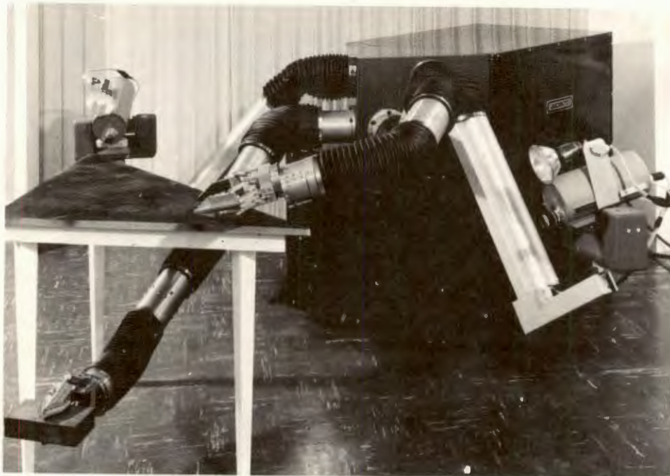
Figure 15. Mobot Mark II with 25-Pound Lead Brick at 5-Foot Arm's Length
