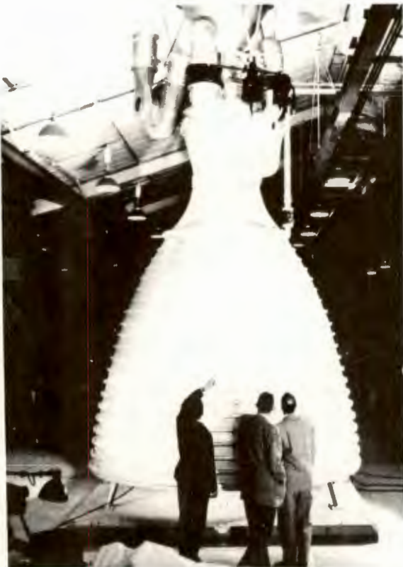
FIGURE 9. SINGLE-CHAMBER ROCKET ENGINE
