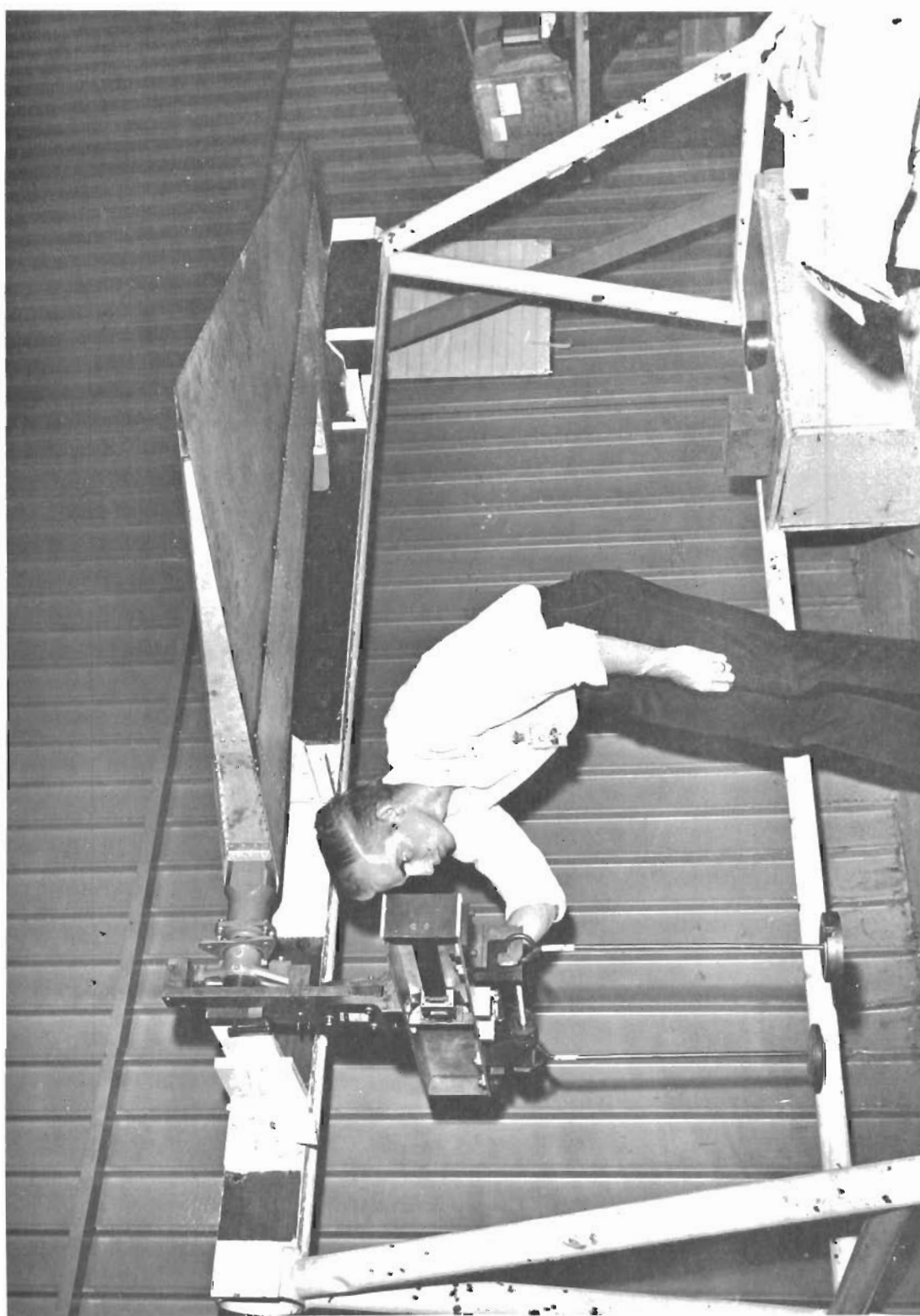
Figure 27 - Mass Balancing of Beryllium Rudder
