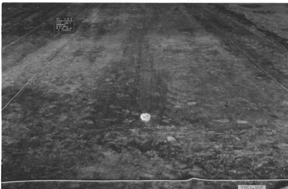
Figure 2. Lane 17 prior to traffic
