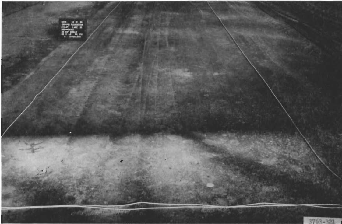
Figure 9. Lane 20 prior to traffic
