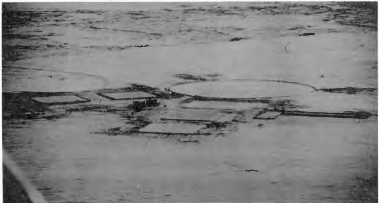
Fig. 4. Aerial view of test site. Square pads are 100 ft X 100 ft. Circular pad is 300 ft in diameter.
