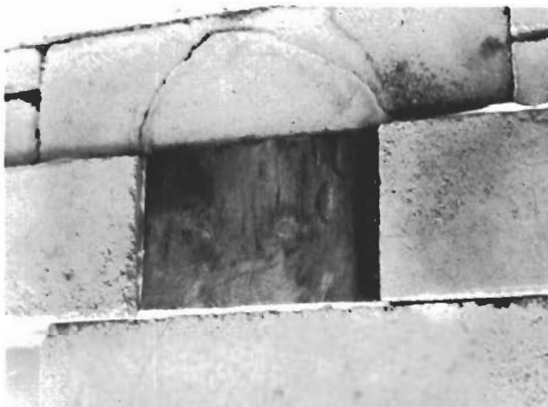
FIGURE 232 - TYPICAL THERMAL TEST SETUP
