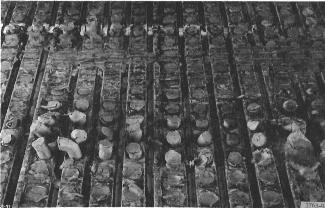
Figure 20. Lane 4, item 2, after two passes of load vehicle, showing extruded soil
