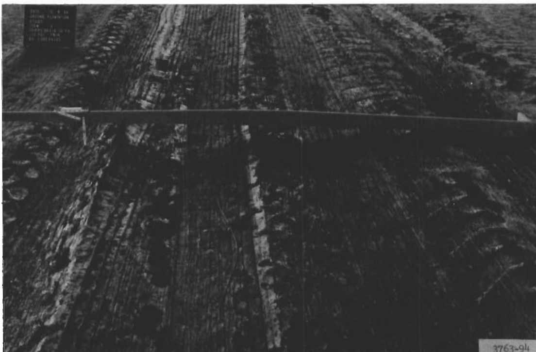
Figure 25. Lane 4, item 3; transverse straightedge shows rutting at 20 coverages (failure)
