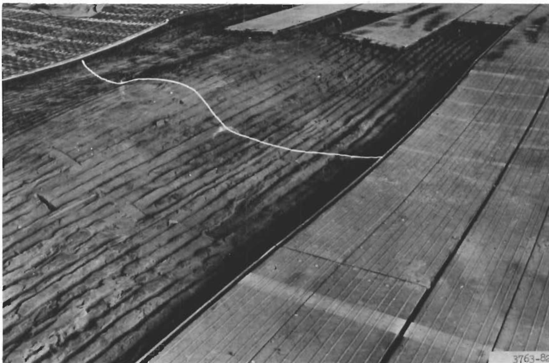
Figure 5. Lane 3, item 1, showing displaced subgrade after mat removal at 458 coverages
