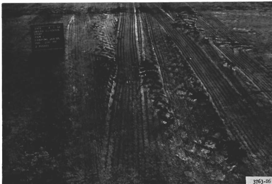
Figure 9. Lane 2, item 1, at two passes (failure)
