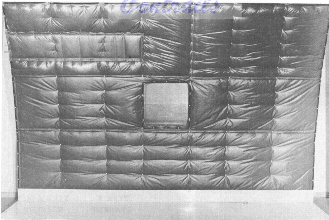
Figure 14. Test Installation of Optimum Blankets - Horizontal Method.
