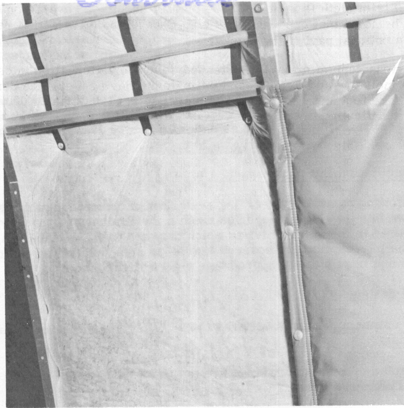
Figure 17. Type Z Blanket Installed on Test Panel.
